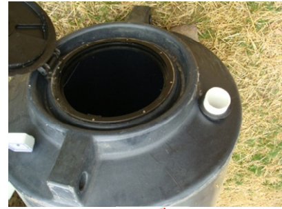
Ring Gasket shown with PVC inlet pipe installed at top of tank
